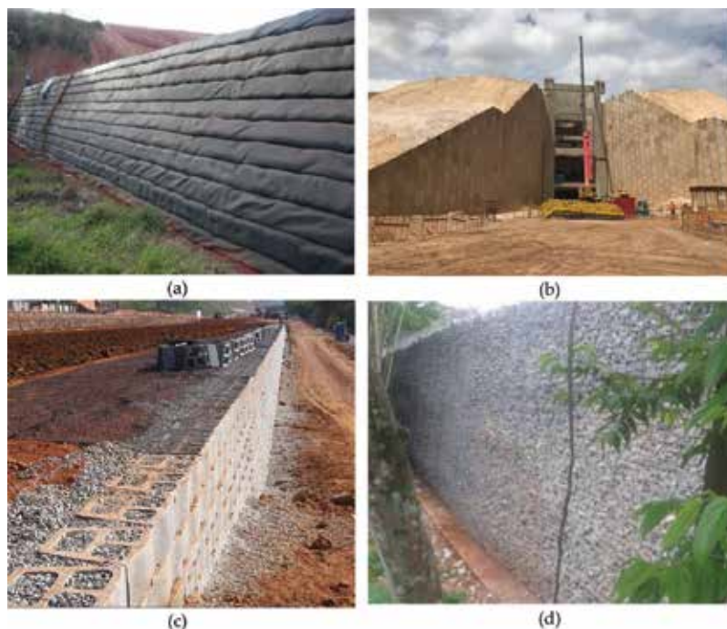
Figure 3. Typical facing elements: (a) geosynthetic wrap-around facing before protection application (courtesy: Ober geosynthetics); (b) precast-concrete panels (courtesy: Reinforced Earth Company); (c) precast-concrete blocks facing; and (d) steel mesh facing filled with stones (courtesy: Paulo Brugger).
