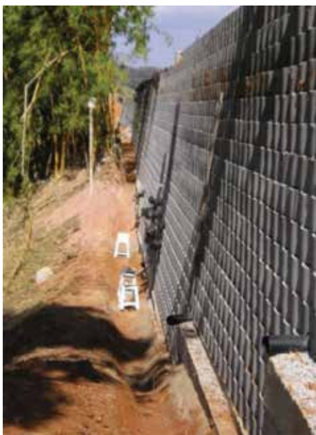
Figure 4. General view of the RSW just after construction.
