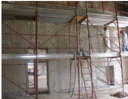
Figure 15. Application of mortar D as the reinforced plaster to Venaria's masonries.
