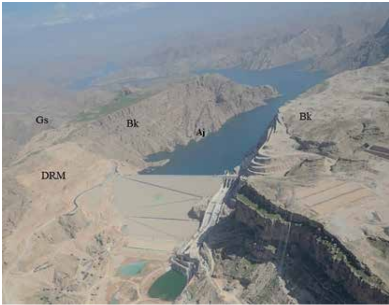
Figure 17. An upstream (eastward) view of Gotvand dam site and the outcropped formations; Bakhtyari (Bk), Agha-Jari (Aj), and Gachsaran (Gs). DRM is displaced rock mass.
