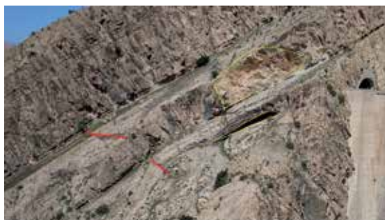
Figure 7. Rock sliding (in yellow) at right abutment of the dam.
