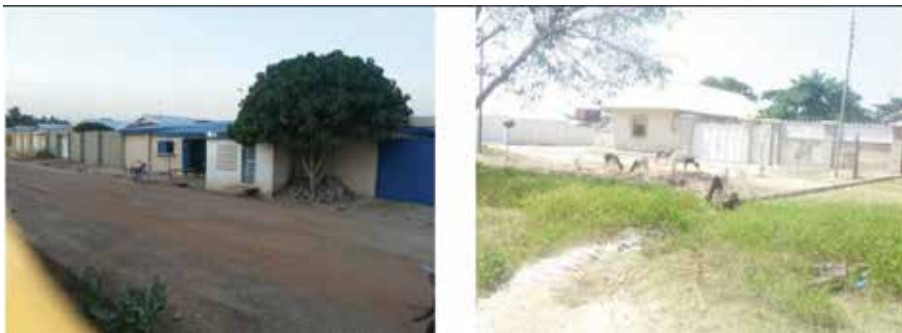
Figure 1. Streets with shops attached to self-built houses in medium-income districts of Katsina and Minna, Nigeria.
