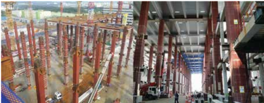
Figure 3. Semiconductor FAB (bolt-connected PSRC composite column).
