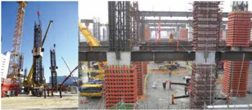
Figure 2. Semiconductor FAB (weld-connected PSRC composite column).
