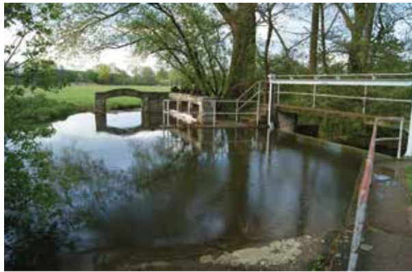
Figure 2. Main sluice (near Mörlheim) along the river Queich (right side of the photo). The sluice is closed which allows water to flow into a main ditch (upper left side of the photo; photo: Martin Alt).
