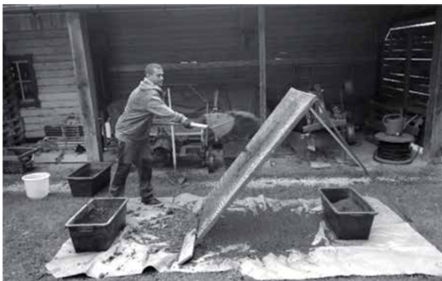
Figure 5. The earth material must be sieved before the boxes are filled (HBLFA Raumberg-Gumpenstein).
