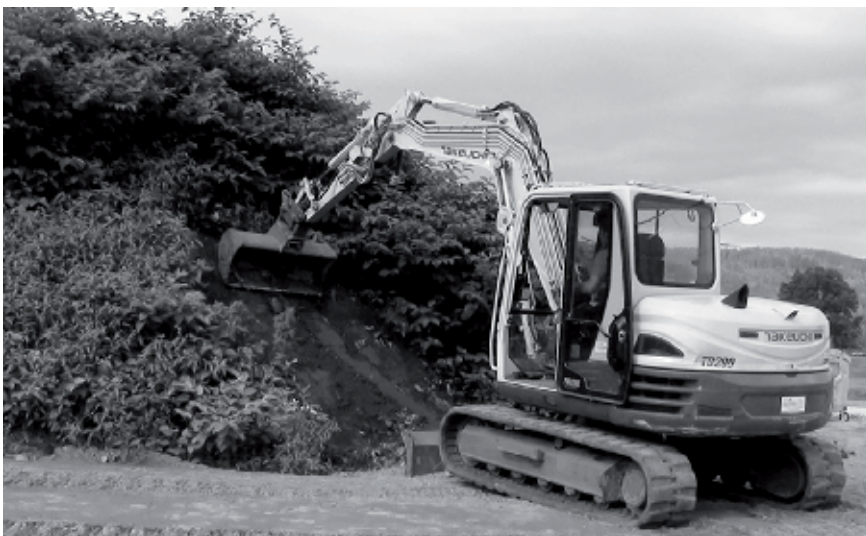
Figure 3. Excavation work at location 1 (E.C.O. Institute of Ecology).
