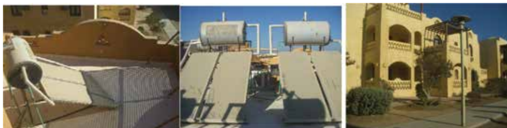
Figure 6. Using solar water heater and PV systems for electricity production in EL Gouna.
