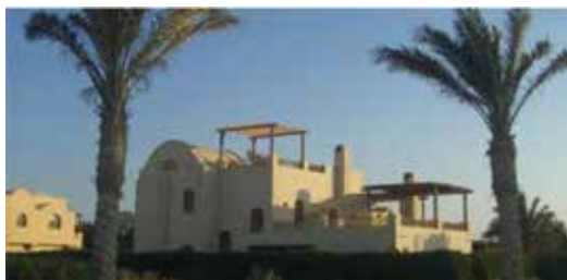
Figure 5. Example for using wind catches as passive cooling strategy in EL Gouna.
