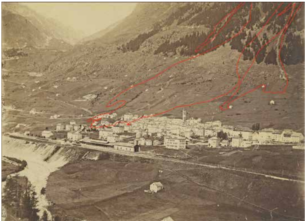
Figure 4. The Sasso Rosso slope failure (Airolo, 1898). Projection of the slide perimeter on an oblique terrestrial image of the area prior to the event (source: Conedera et al. [21]).
