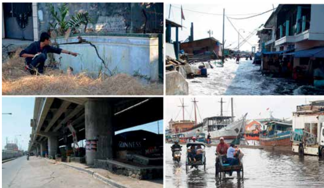
Figure 6. Pictures of the impact of subsidence (e.g. cracks in buildings and infrastructures and tidal inundation) in Jakarta, Bandung, and Semarang (source: authors).
