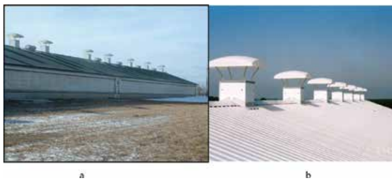
Figure 2. Naturally ventilated (a) pig finishing building with (b) close-up of modern controlled ridge vents.
