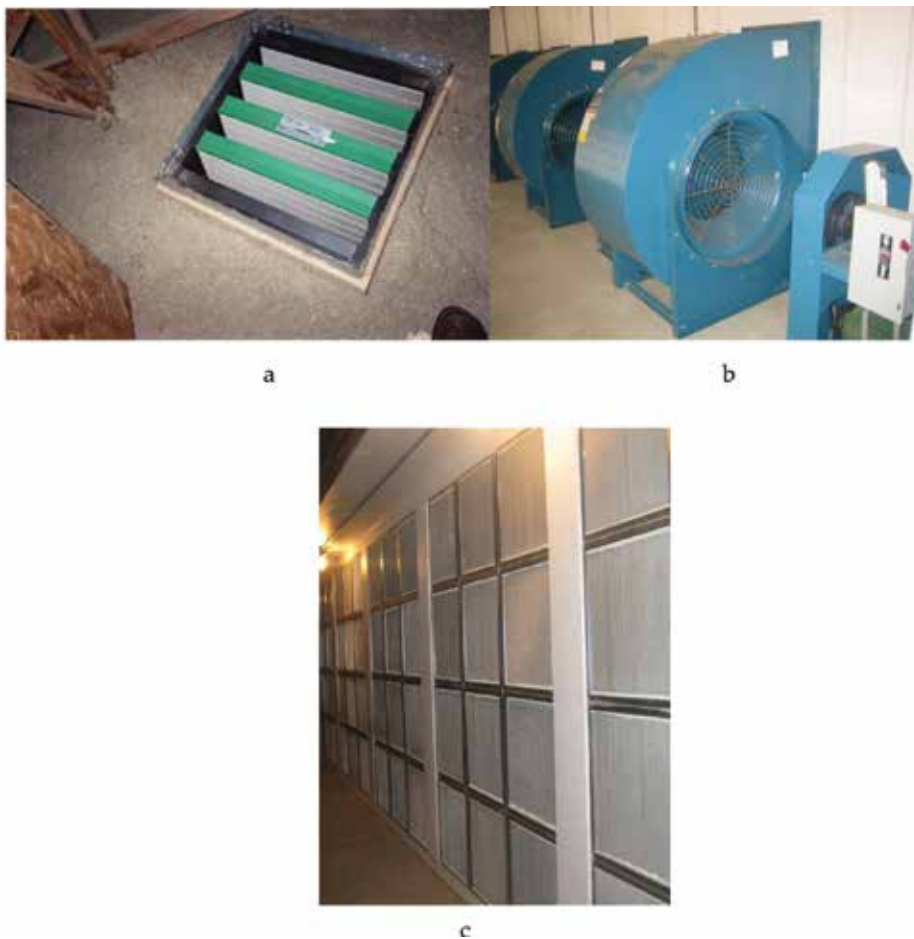
Figure 8. Virus filtration with (a) filters attached directly to ceiling fresh-air intakes in a negative pressure system, or (b) using blowers and (c) filtration banks in a positive pressure filtration system.
