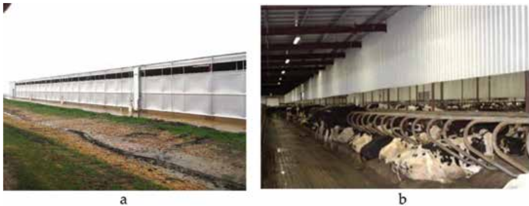
Figure 7. (a) Dairy housing sidewall inlet with or without evaporative cooling pads and in some cases (b) drop curtains/walls to force cross-flow ventilation over rows of cows, enhancing airspeed maintenance.
