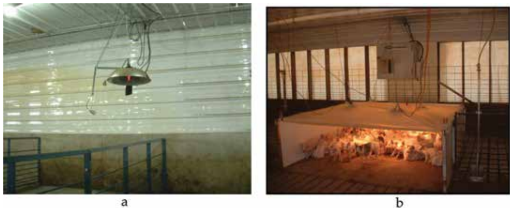
Figure 5. (a) Radiant spot heater with shielded radiant sensor for feedback control and (b) microclimate with heat lamps.
