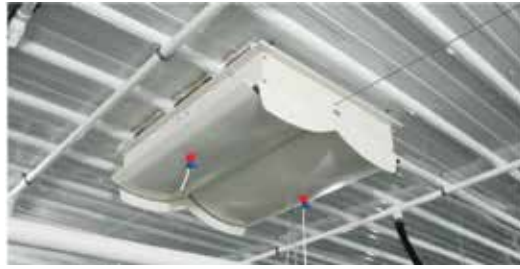
Figure 4. Example ceiling fresh-air diffuser commonly used in HLPP systems. The cable shown passing through the diffuser is used to automatically control baffle opening in response to ventilation rate changes with static pressure control as the ultimate diffuser opening control objective.
