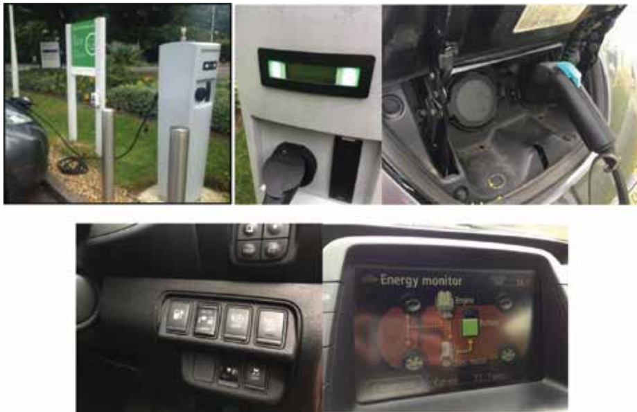
Figure 6. (a)–(e). On-site WPC facilities and charging compatibility.
