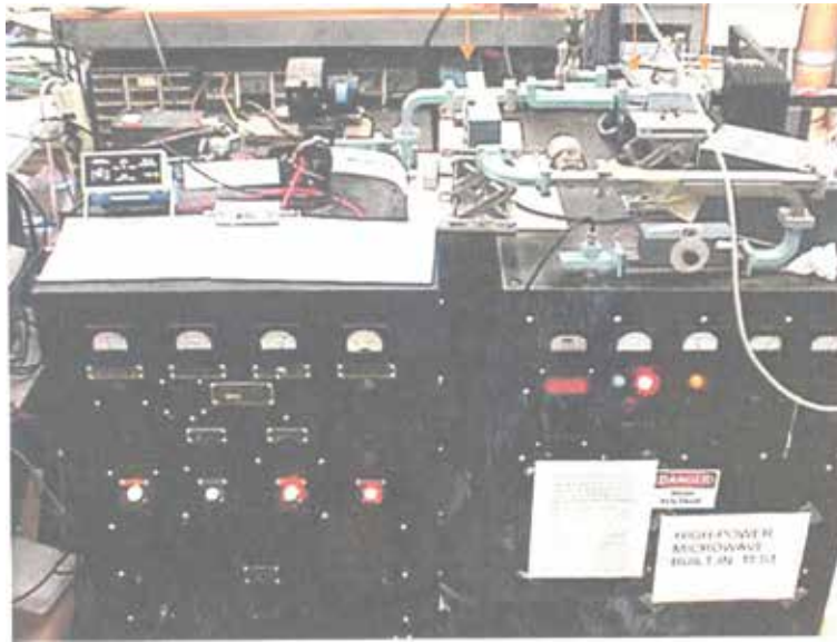
Figure 5.8. Magnetron (center) with waveguide (right) on the top of power supply and pulser cabinets.
