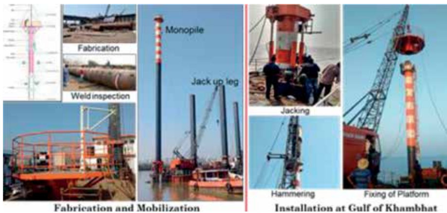
Figure 5. Installed LiDAR at Gulf of Khambhat for MNRE-NIWE.
