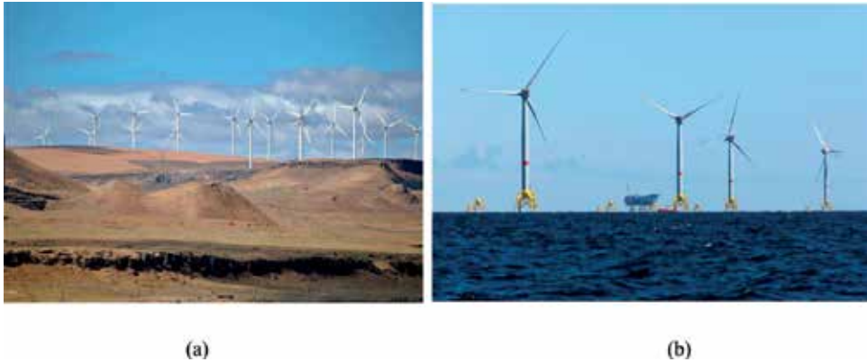
Figure 8. Onshore and offshore wind farms.
