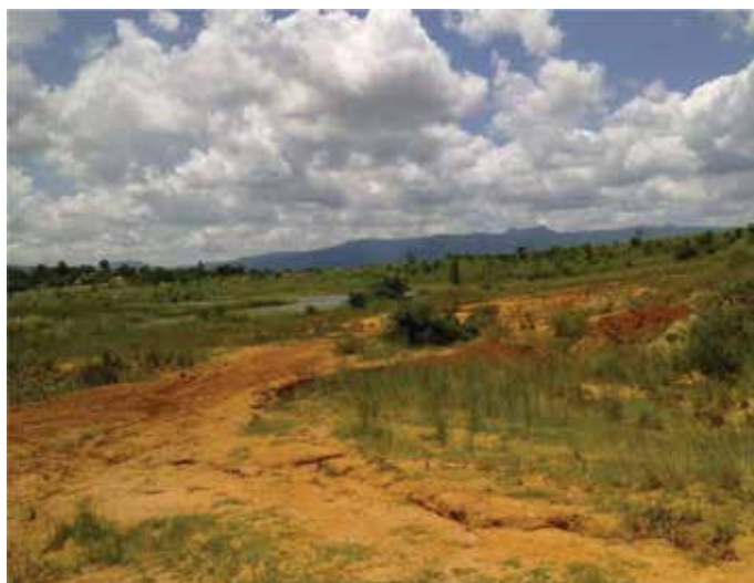
Plate 1. The defunct Mambedi dam after the 2000 floods (December 2008).
