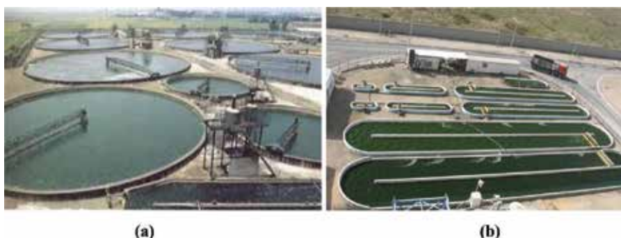
Figure 1. Open ponds cultivation system of microalgal cells. (a) Circular open pond and (b) raceway pond.
