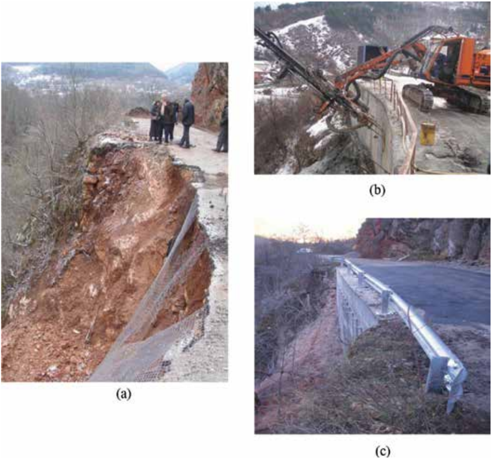
Figure 10. (a) Road breakage; (b) stage of repair; (c) ready road.
