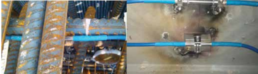
Figure 14. Installation diagram of FBG temperature sensor.
