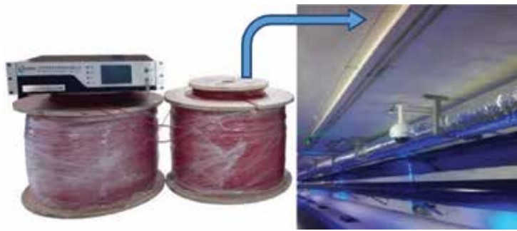
Figure 10. Application of the DTS system to fire monitoring in urban underground comprehensive pipe corridor.
