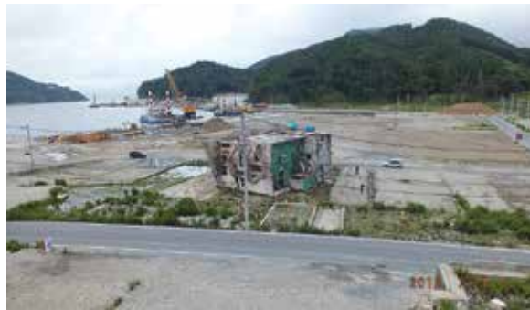
Figure 20. View of disaster site (Onagawa-cho, 28 months after the event) (photo by Daigoro Isobe).
