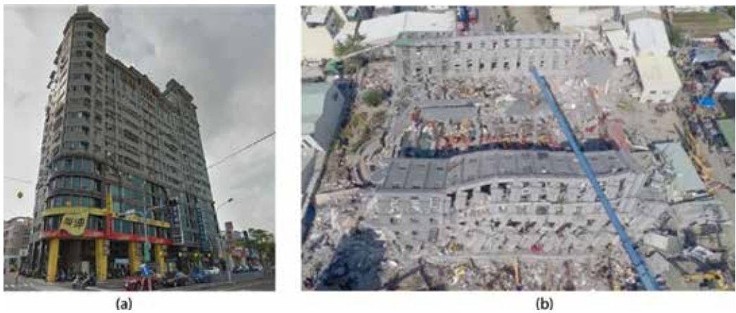
Figure 9. The Weiguan building: (a) before the collapse [11]; (b) after the collapse [13].
