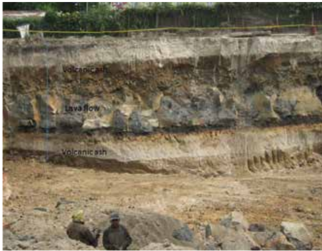
Figure 14. Interbedding of lava flow and volcanic ashes in San Salvador City (see location in Figure 1a).
