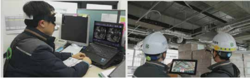
Figure 2. Improving BIM with gear VR glasses in a desktop and in a work place [18].
