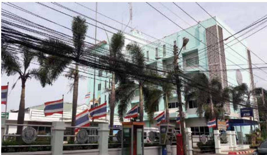
Figure 7. Kho-hong municipality office.
