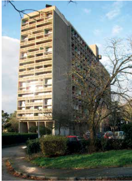
Figure 13. This is an image of the le Corbusier structure in Rezé-Nantes. This building is popular for artists and architect to live within — Copyright © 2012, Jon Bryan Burley, all rights reserved, used by permission.
