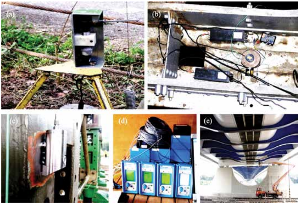
Figure 10. Examples of bridge DLT instrumentation: (a) inductive displacement transducers (IDT); (b) accelerometers set up; (c) strain sensor (d) charge amplifiers devices; (e) accelerometer installation process to bridge bottom for DLT.
