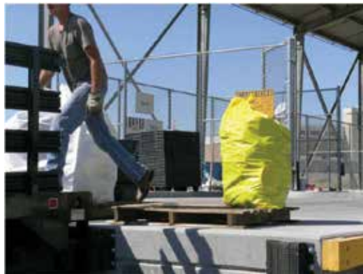
Figure 15. Before intervention, off-loading truck at sorting area.
