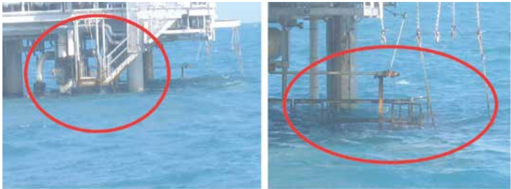
Figure 2. Subsidence evidence on oil and gas platform offshore.
