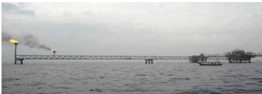
Figure 1. Oil and gas platform offshore.
