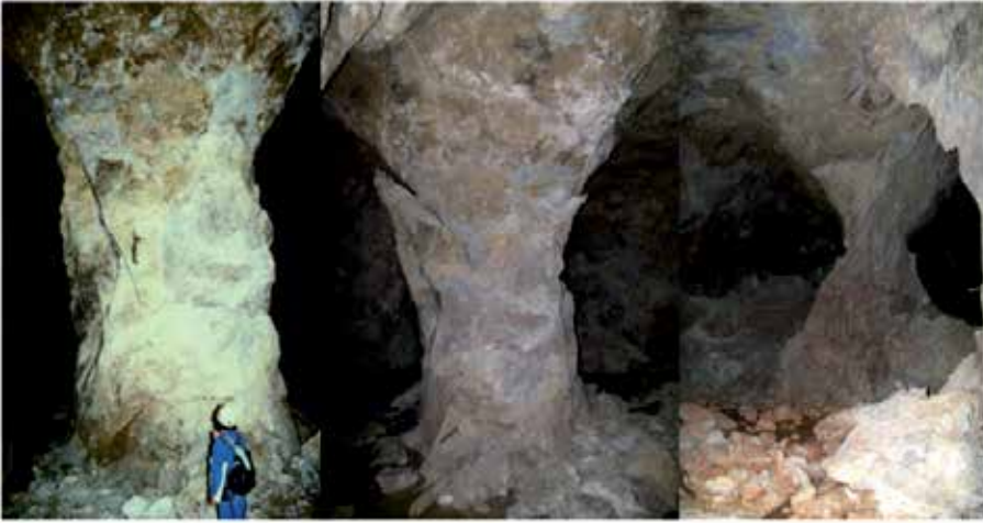
Fig. 7. Progressive spalling of a pillar in a gypsum mine. From left to right, photos from 1996, 2000, and 2004 (Sorgi & Watelet, 2007)
