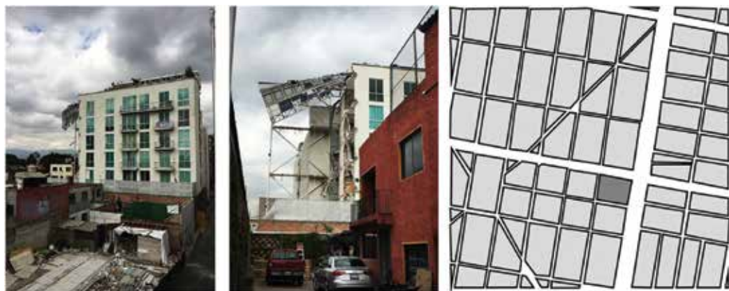
Figure 3. Collapsed buildings in Mexico City in the September 2017 earthquake. Despite the density of the buildings, the absence of public space in the surroundings is evident. Photo: Rosa Lilia Pedraza Vázquez.
