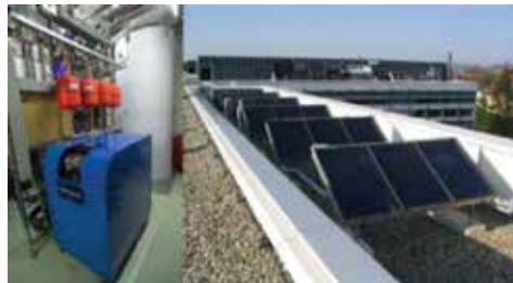
The Fraunhofer ISE institute building and SorTech adsorption chiller in the technical room (sources: Fraunhofer ISE) [34]
