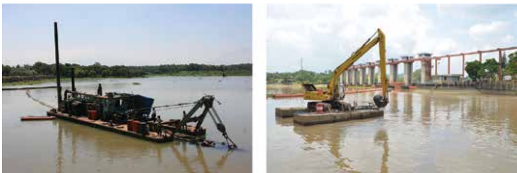
Figure 10. Sediment dredging works in Wlingi reservoir (left) and Lodoyo reservoir (right).
