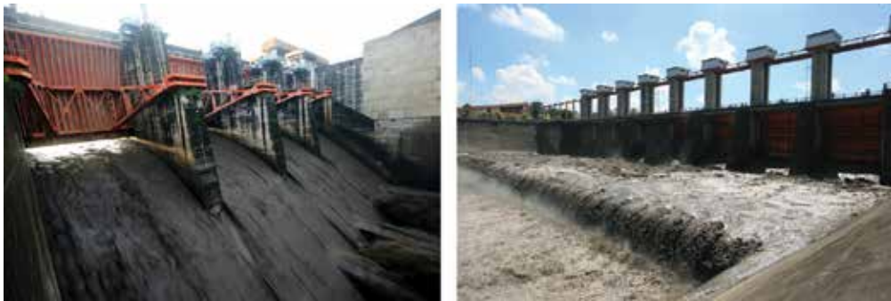
Figure 11. Sediment flushing through spillway gates in Wlingi reservoir (left) and Lodoyo reservoir (right) on 29–31 March 2013.
