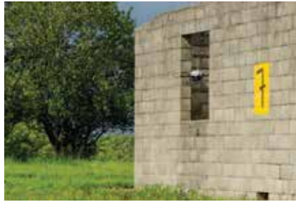
Figure 19. Indoor rotorcraft entering the building via broken window (source: ICARUS).
