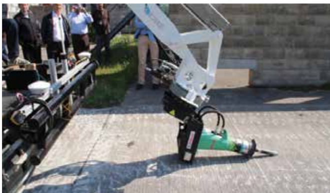
Figure 15. The jackhammer is being attached to the arm of the LUGV (Source: ICARUS).
