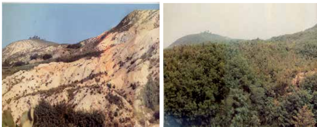
Fig. 3. Before and after the construction of a hillside planting work in South Korea
