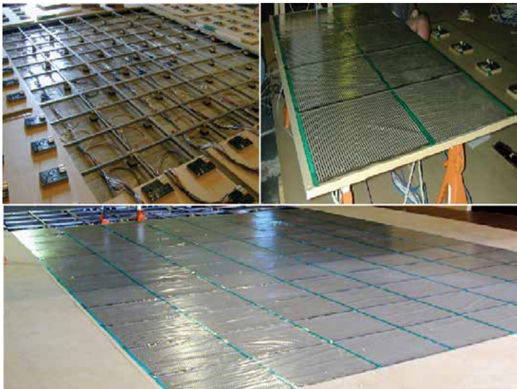
Fig. 1. Sub-floor steel framework (top left), surface floor wooden framework (top right), Complete view of AME Floor-III after assembly (bottom).
