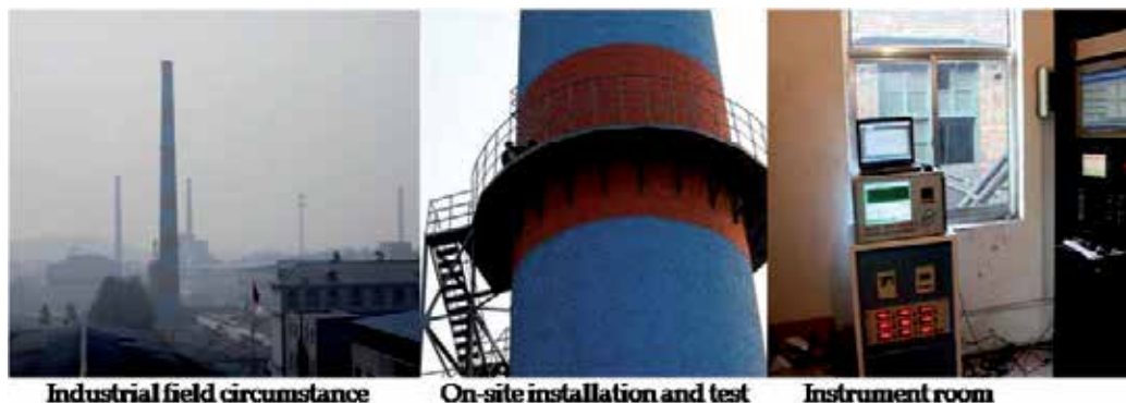
Fig. 16. One of the testing circumstances for in situ on-line monitoring of industrial emissions.
