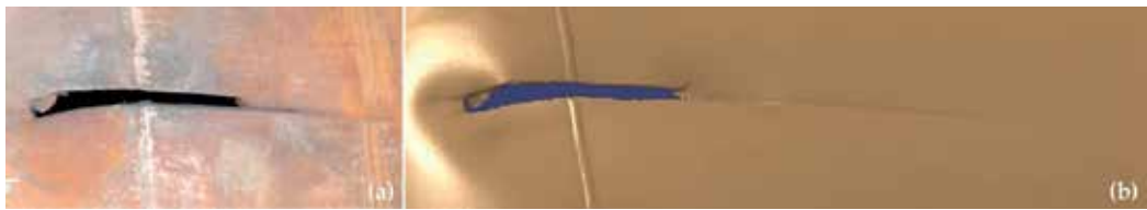
Figure 30. (a) Photograph of the cut present on the tank shell of carriage no. 1 and (b) digital model of the cut obtained by reverse engineering reconstruction based on geometry acquisition with a time-of-flight laser sensor.
