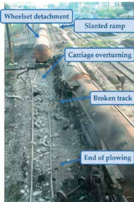
Figure 7. Superstructure zone wrecked due to the “plowing” mechanism of the track by the front wheelset of the first bogie.
