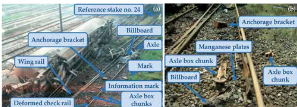
Figure 24. Zone of the heart of railway switch 13B around the wing rail and the check rail immediately after the accident.
