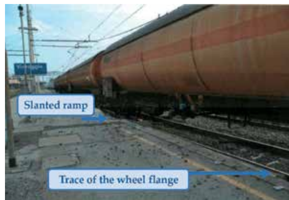
Figure 5. Walkway at grade endowed with a slanted ramp on the sidewalk, near the track of the derailed train, and trace on the granite curb left by the flange of the right wheel of the front wheelset of the first bogie of carriage no. 1.
