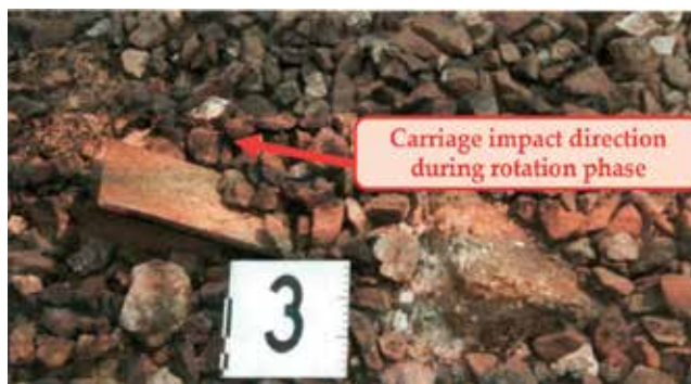
Figure 17. Track reference stake no. 23, photographed during the investigations on the accident site conditions, partially buried in the track ballast following its impact against the pressure vessel of carriage no. 1.
