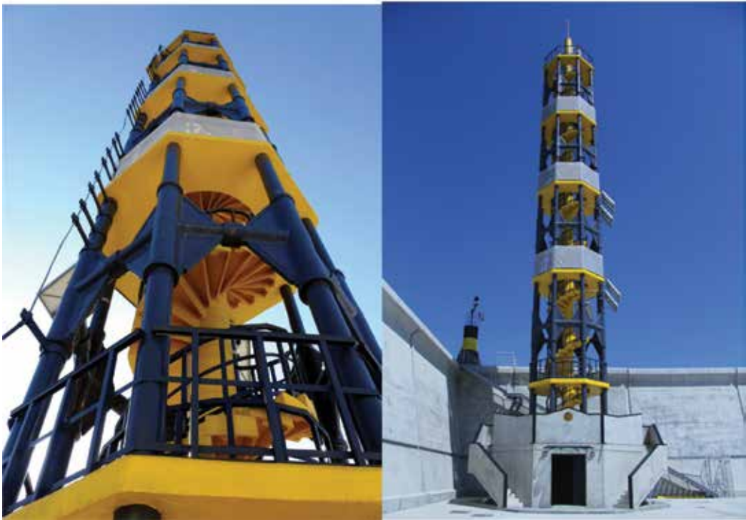
Figure 8. The FRP lighthouse (Valencia, Spain): Left: lighthouse detail, Right: general view of the lighthouse in Port of Valencia.
