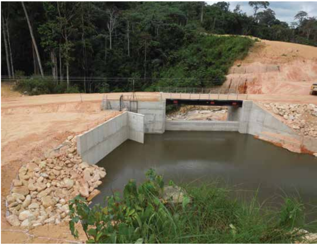
Figure 5. Iboundji bridge (Gabon, Africa).
