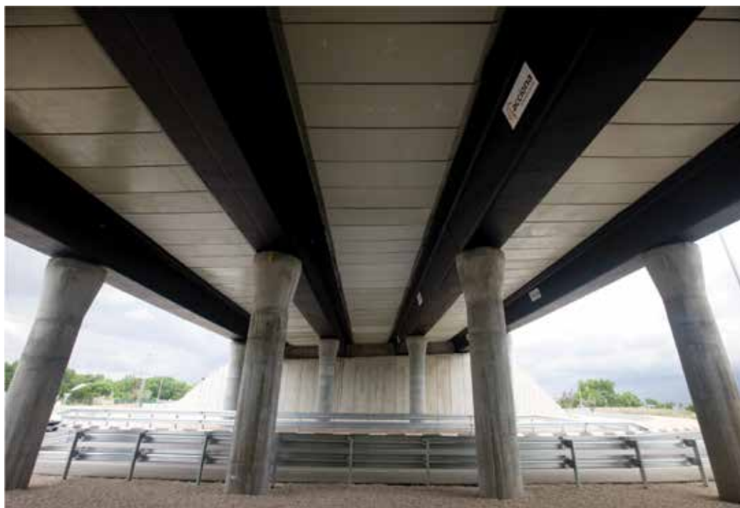
Figure 4. M111 bridge (Madrid, Spain).
