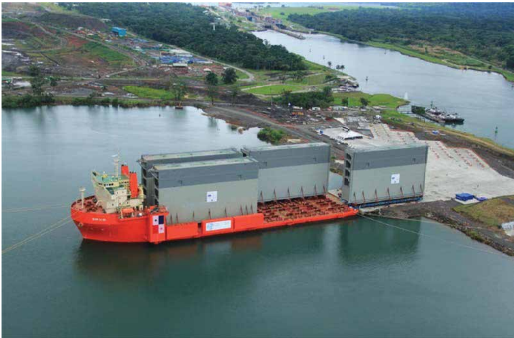
Figure 11. Unloading of the gates on the quay side Atlantic.
