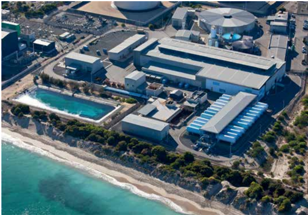
Figure 5. Perth desalination plant.
