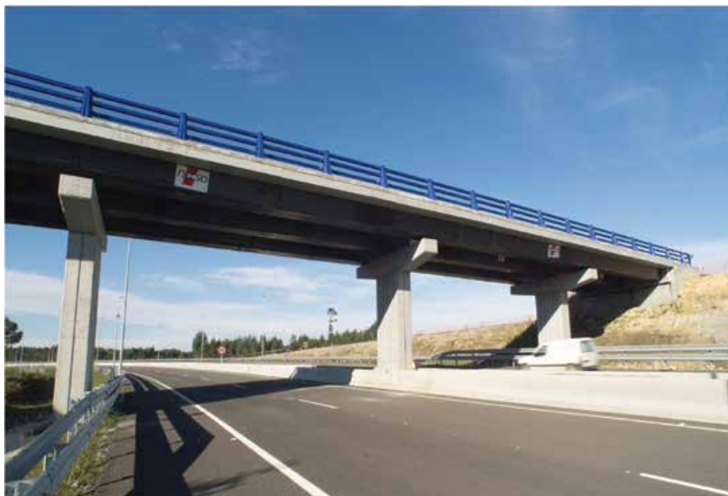
Figure 2. Composite bridge in Asturias (Spain).
