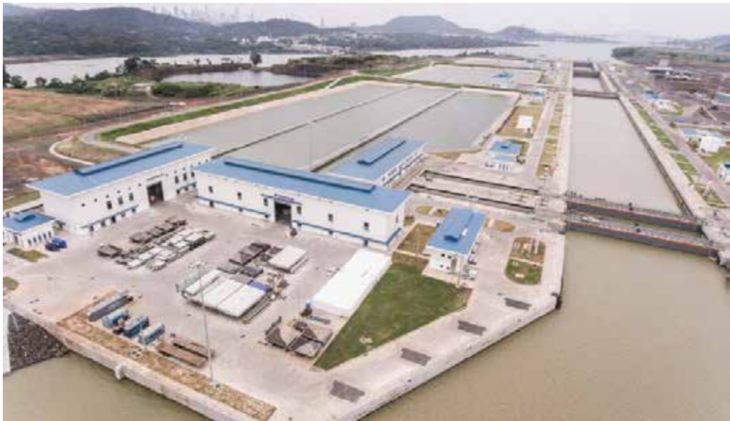
Figure 10. Overview of the structure where the two gates are located at each end of the chamber.
