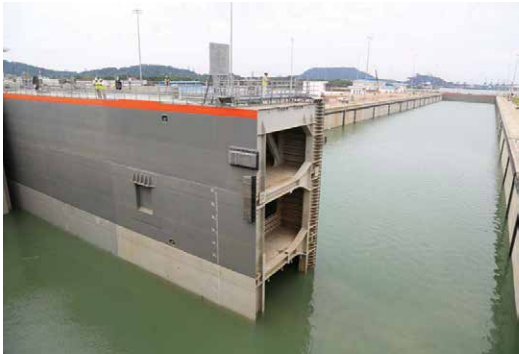
Figure 9. Overview of a gate in operation.
