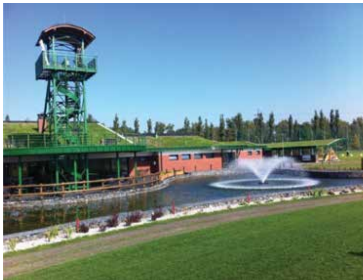
Figure 7. Golf club building at undermined territory.
