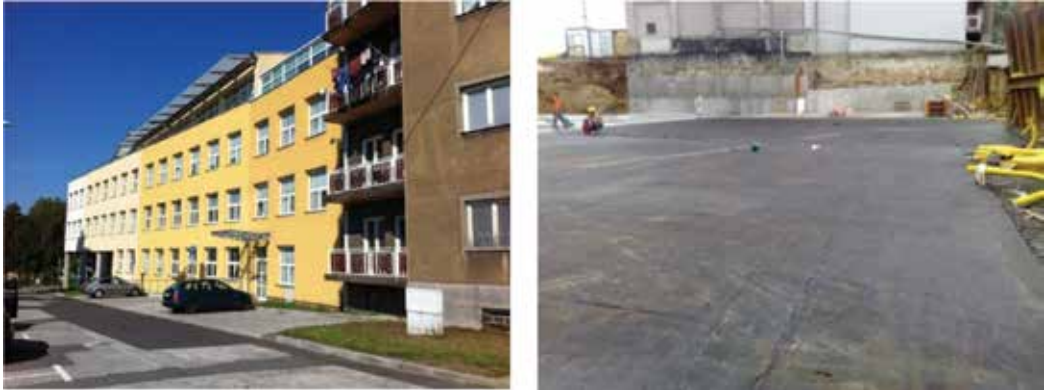
Figure 6. University of Ostrava Building, application of sliding joint.
