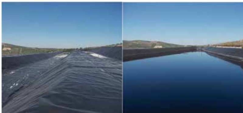
Figure 1. Ponds for the confinement of the wastewater (left = before filling, right = after filling) from the extraction of olive oil at the facility of Coop. Sor Ángela de la Cruz, Estepa (Sevilla, Spain). Due to the environmental toxicity of the liquid phase, the large amounts produced from intensive olive tree cultivation in that area need to be stored separately before further processing, e.g. for biogas production (Source: Marco Nuti).
