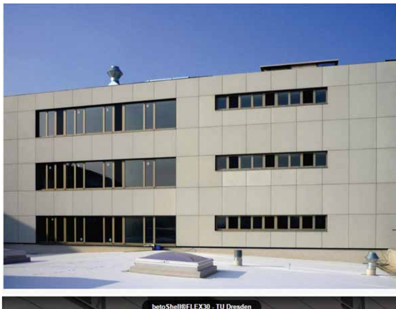
Figure 13. бетоShell© façade application developed by Hering Bau [95].
