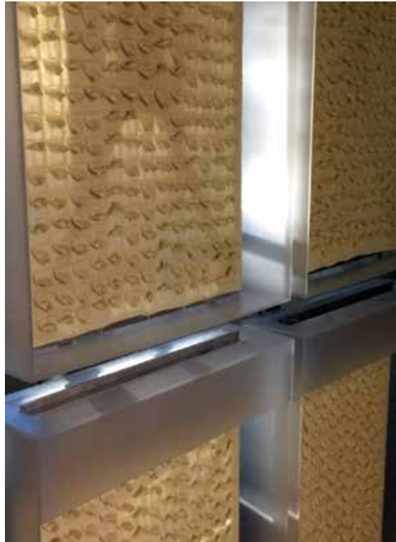
Figure 11. Close up of FELT Plexiglas frames and textile panels.
