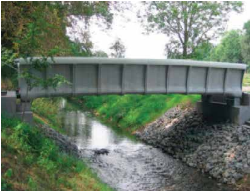
Figure 12. First segmental TRC Bridge in Oschatz, Germany [94].
