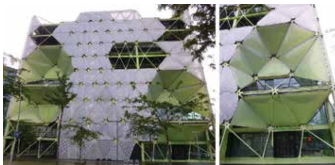
Figure 10. Media-TIC building: (left) exterior view and (right) inflatable cushions [40].
