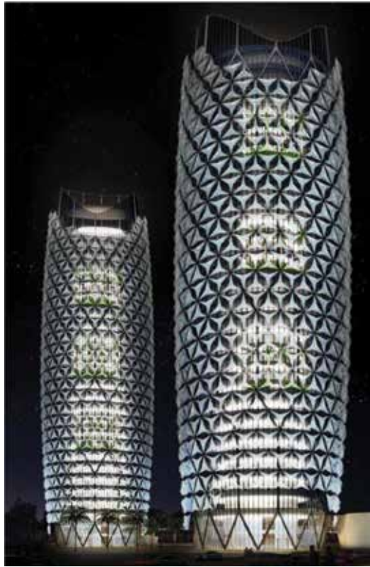
Figure 8. Abu Dhabi Towers (taken from ihabitat.com).
