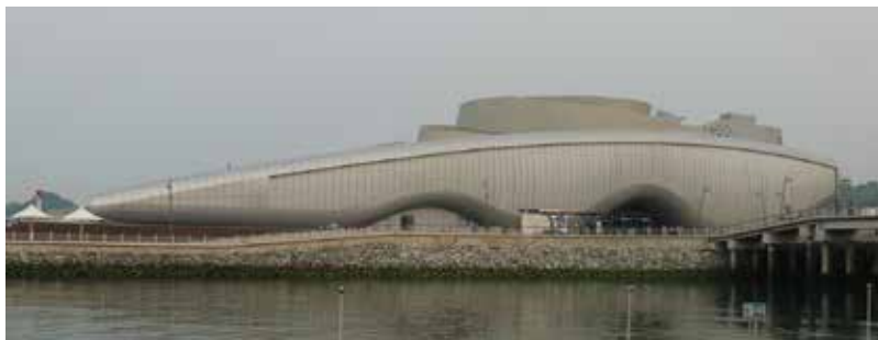
Figure 13. The kinetic façade and closed lamellas [47].
