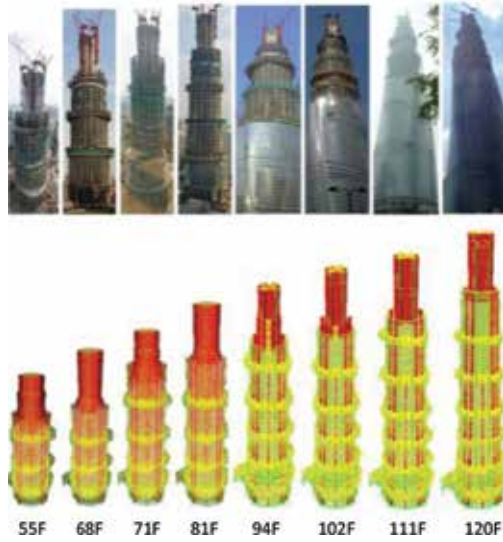
Figure 11. Overview of buildings in different stages and finite element models, field test on a typical floor.
