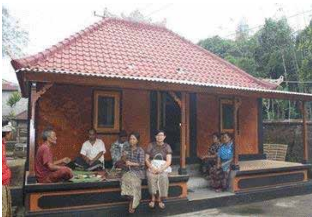
Figure 10. The simple traditional Bali age house with the bamboo reinforced concrete structure and brick walls [23].
