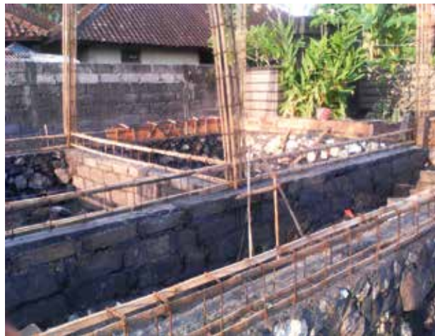
Figure 9. The bamboo reinforcement was assembled before concrete was casted [24].
