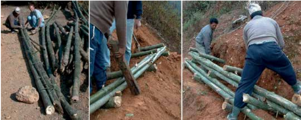
Figure 1. Crib wall construction steps in Thankot (Nepal) 2002 [7].
