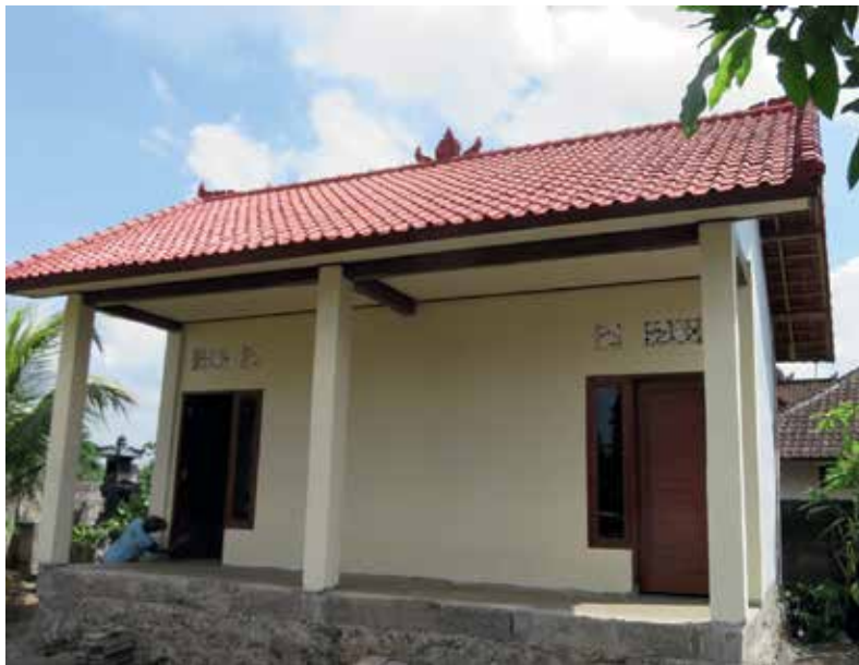
Figure 12. The simple modern Balinese house with the bamboo reinforced concrete structure and concrete block wall [24].
