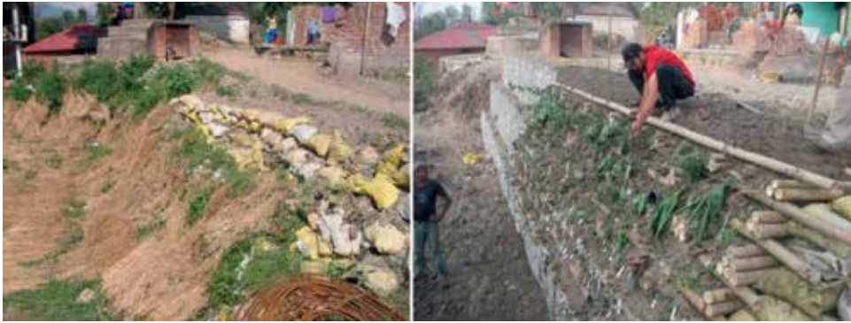
Figure 6. Before and after construction photographs, Kusunti, Lalitpur (November 2007) [26].
