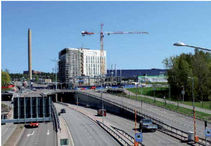
Fig. 11. Photo of the Skanska building partly ready.
