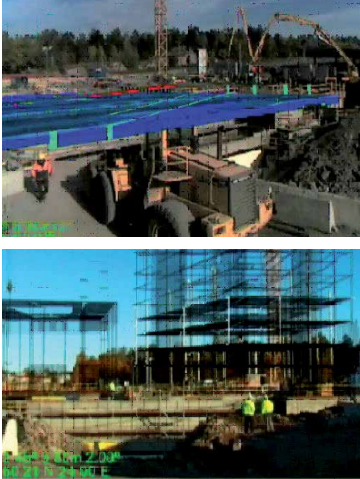
Fig. 10. Mobile AR during construction work.
