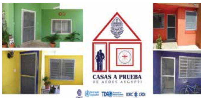
Figure 1. Photographs show Aedes aegypti -proof houses with insecticide-treated screens mounted on aluminium frames and fixed to external doors and windows of treated houses.
