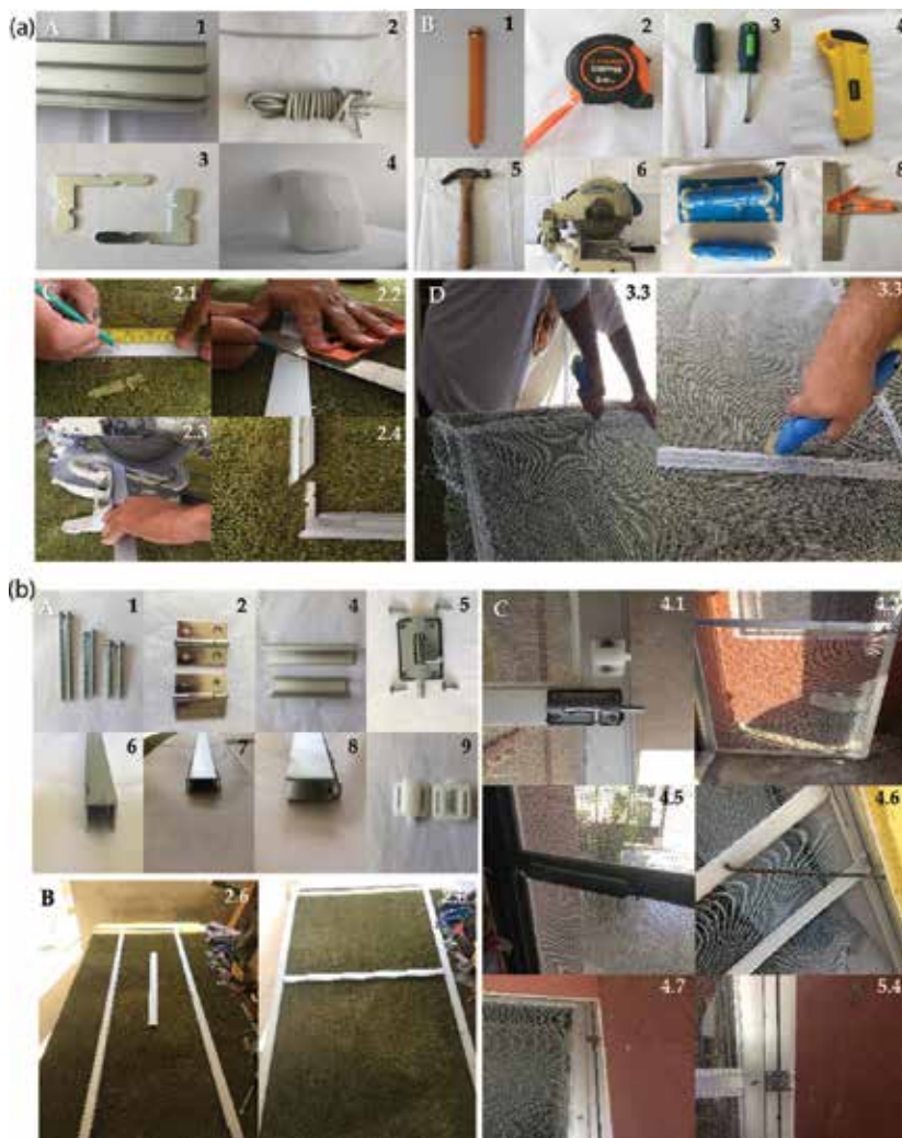
Figure 2. General description of how to install insecticide-treated screens on windows and doors. Window: (A) Materials required: (1) screen frame, (2) square for screen frame, (3) vinyl #12 and (4) window screen. (B) Tools required: (1) pencil, (2) measuring tape, (3) screwdriver, (4) sharp knife, (5) hammer, (6) hacksaw, (7) convex wheel and (8) universal square. (C) Step 2: (2.1) Using a measuring tape and pencil, make a mark where a cut is to be made on the new frame. (2.2) With the universal square, mark a 45° angle on the first mark of the final measure. (2.3) Use the hacksaw to make the 45° cut. Make four cuts, one on each side of the window. (2.4) Use squares to join the four parts of the frame. Insert squares into the frame along the side with 45° cut and lightly tap the squares into place. Check the assembled frame for squareness. (D) Step 3: (3.3) With the help of the convex wheel, insert the screen into the channel with vinyl, beginning at one corner (press down and roll with short strokes back and forth). When all sides have been inserted into the vinyl, remove the excess vinyl. Door: (A) Materials required: (1) screws (1 ½ × 8", ½ × 8, 1 × 8), (2) hinges, (3) vinyl # 12, (4) elephant trunk handle, (5) hasp, (6) chair butt, (7) mosquito door frame central, (8) mosquito door frame vertical and (9) lock. (B) Step 2: (2.6) Forming the door, 1 ½ × 8 screws should preferably be used. Step 4: (4.1) The lock and pin are installed in the central part of the frame, at the appropriate distance for its correct operation. (4.2) The elephant trunk handle is installed in the central part of the frame. (4.5) Spring allows the automatic closing of the door. (4.6) Pivot allows the automatic closing of the door in a slow and controlled way. (4.7) Metal mesh protects the mosquito net from damage caused by animals. Step 5: (5.4) Fix the door to the frame using ½ × 8 screws, a drill and a screwdriver. Check the assembled door for squareness.
