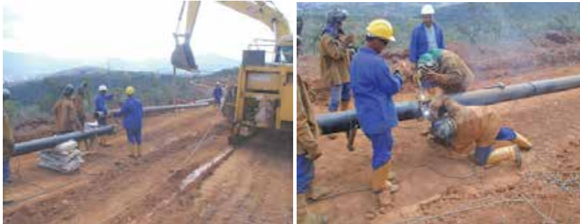
Fig. 29. Preparation of a pipeline assembly. (a) pipes positioning and (b) root pass.
