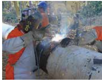
Fig. 30. Pipeline manual welding procedure.
