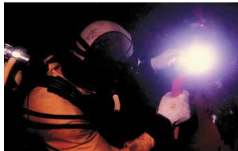
Fig. 2. Underwater welding with SMAW.
