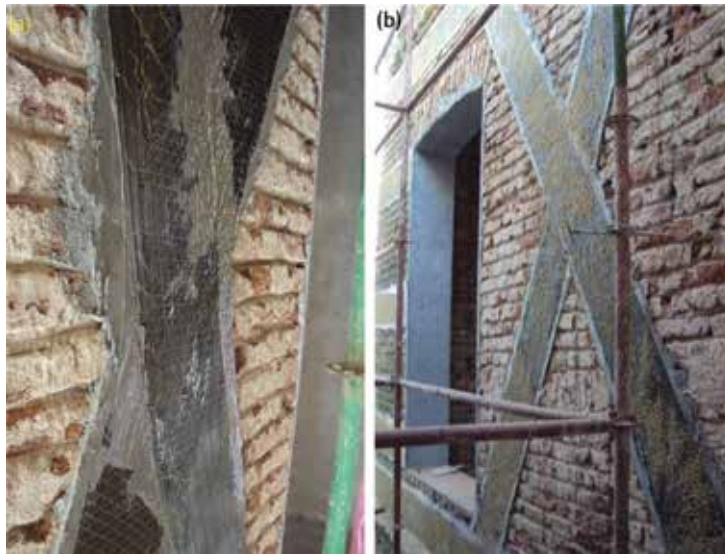
Figure 4. Carbon fiber wrap applications on masonry walls (a and b).
