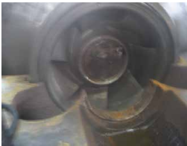
Figure 2. Failure scenario of the centrifugal pump showing the fractured rotor shaft.
