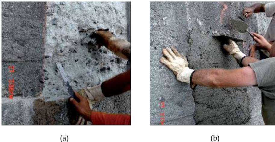
Fig. 10. (a) Application of bridge bonding. (b) Launch of the repair material.
