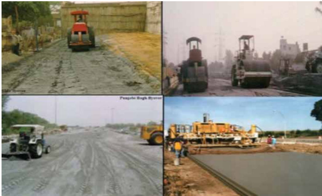
Figure 17. Utilization of fly ash in different road.
