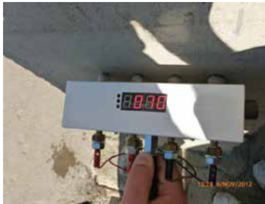
Figure 8. The measurement of a concrete pillar, first measurement.
