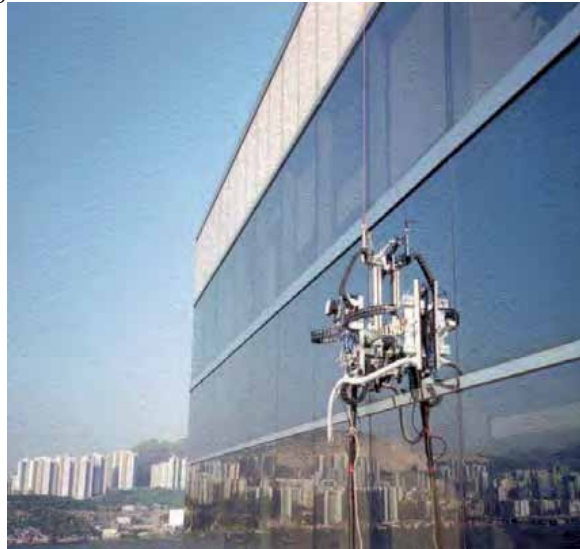
Fig. 3. The climbing robot on site trial outside a commercial building (provided by BBC)
