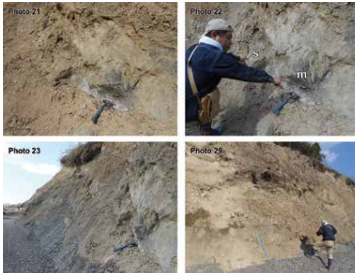
Figure 3. Example photographs of the fracture zone described in Figure 2 . Photo 22 shows mudstone (right; m) and sandstone (left; s) chaotic blocks in the fracture zone.
