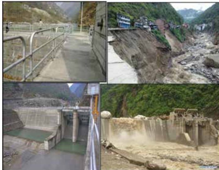
Figure 4. Impacts of GLOF of hydropower UBHP (45 MW), July 2016.
