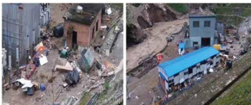
Figure 3. Flooding washed way Bhotekoshi Hydropower Project, July 6, 2016 4:11.
